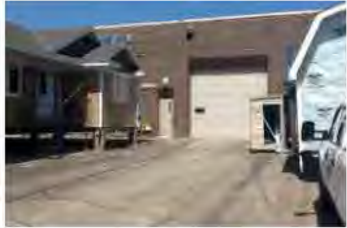
View of south side of the building outside D84 Carpentry
