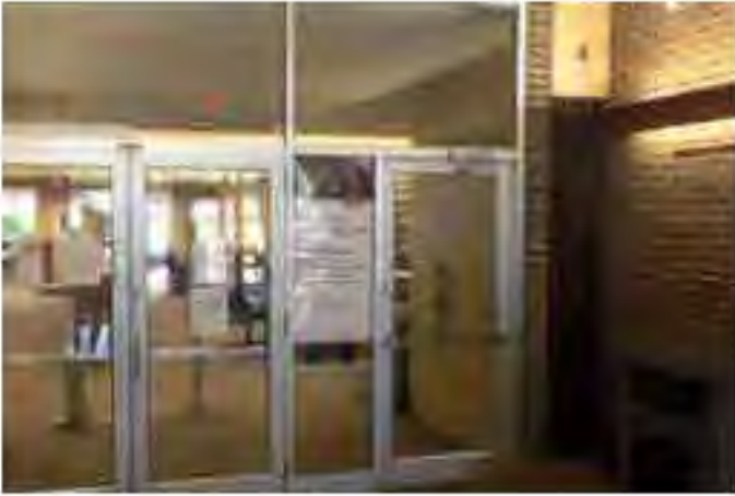
Landing inside main entry
