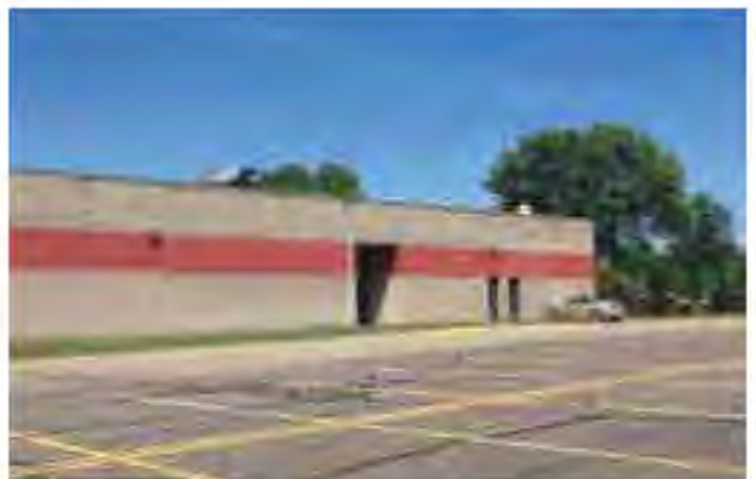
View of secondary entry on south side of building
