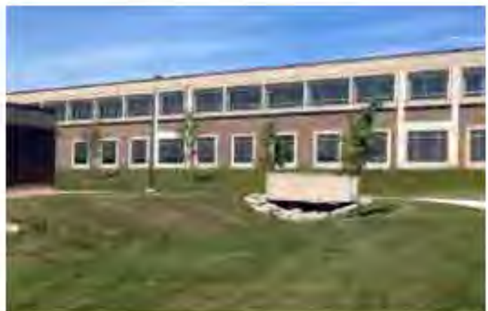
View of southeast side of building
