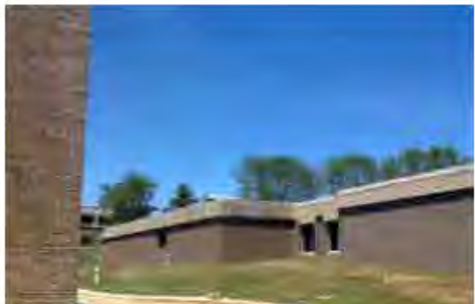
View of southwest side of building
