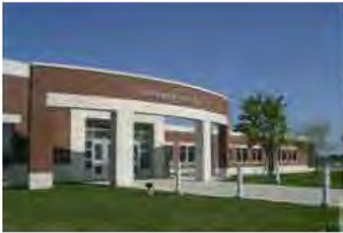
View of current main entry on west side of building
