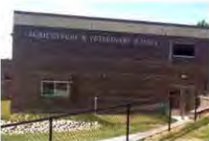
View of main entry on northeast side of building
