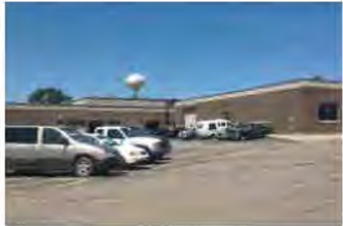
View of southeast side of the building looking northwest
