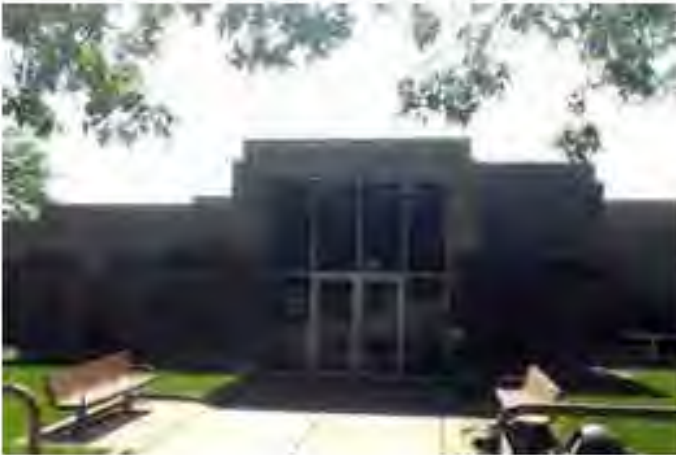
View of current main entry on southwest side of building facing quad
