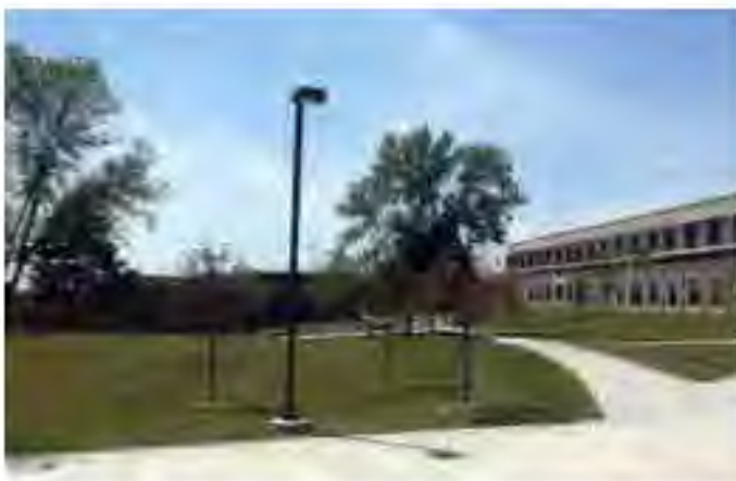
View of southeast side of the building facing primary open space
