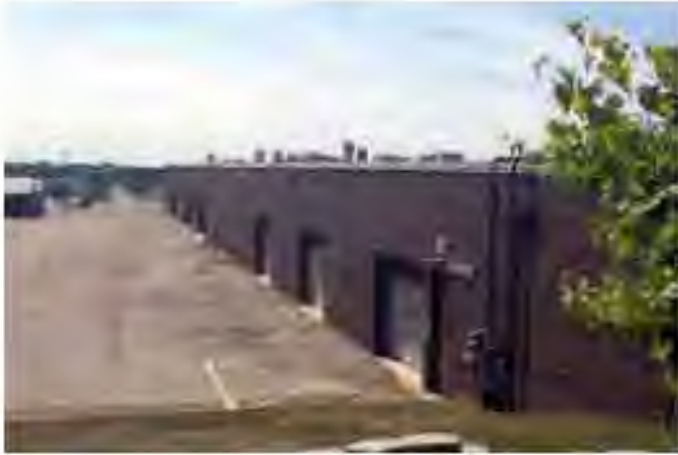
View of east side of building
