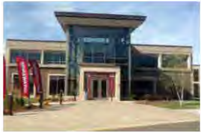
View of current main entry on northeast side of building
