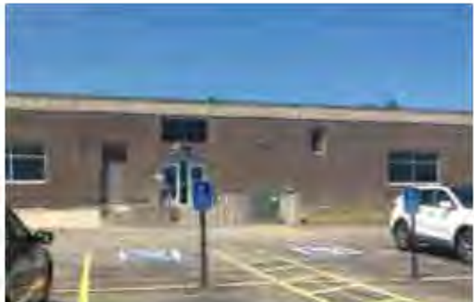
View of southwest side of building
