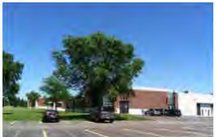
View of southwest corner of building
