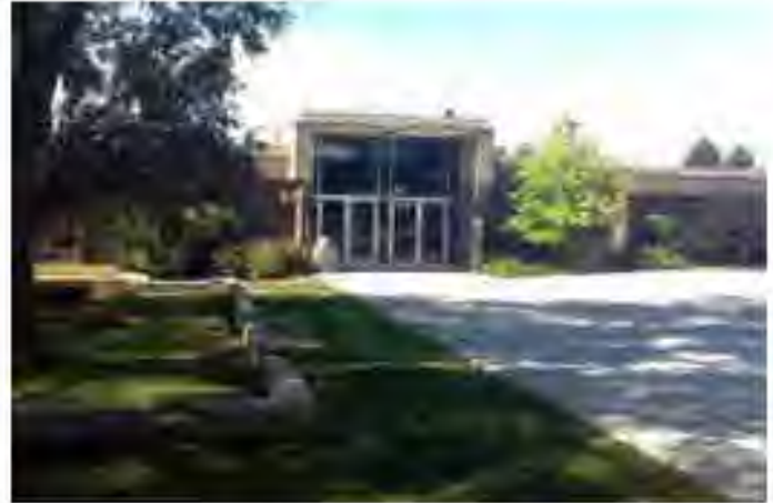
View of entry looking southwest
