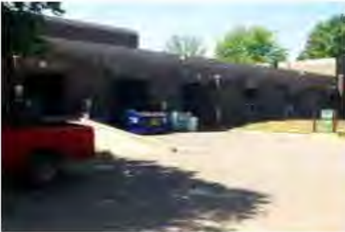
Loading/ service area adjacent maintenance space on main level northeast side
