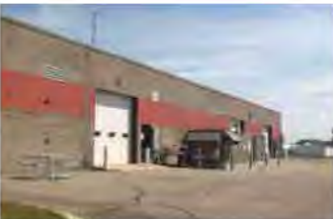
View of overhead doors on west side of building
