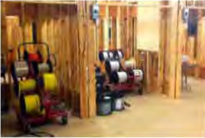
D197 Electrician Program Main Level
