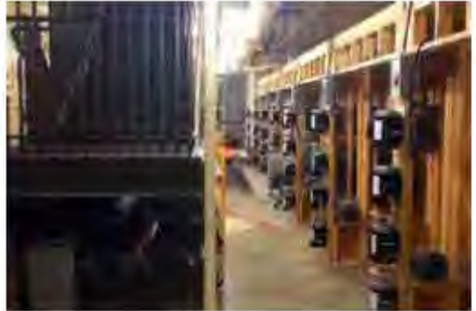
D86 Electrician Program Lower Level
